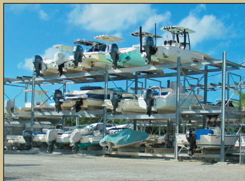
70 Dry Storage Racks
